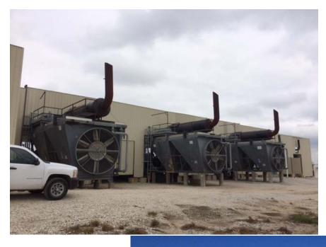
Engine exhaust piped out or set with cooler/exhaust outside
